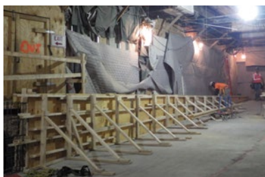
型枠合板(輸出先での使用例) Formwork-purpose plywood (example of use in an importer country)
